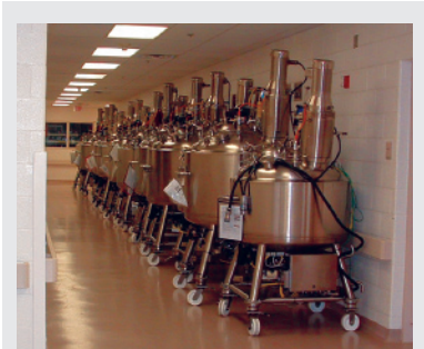
Portable Vessels for Eyewash Batching
