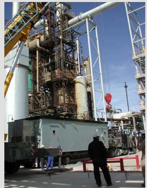
RIE Being Lifted into Place at Refinery
